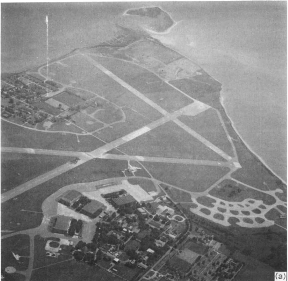
Fig. 2a. Aerial view of trials site.
